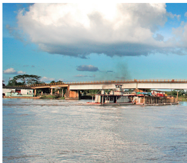
Bridge over the Meta River, Puerto López
